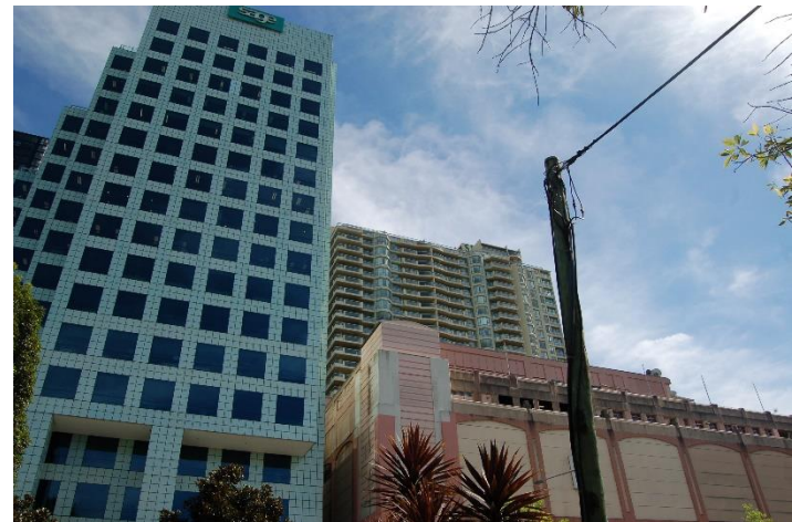
THE SITE LOOKING NORTH EAST FROM CHATSWOOD PARK
